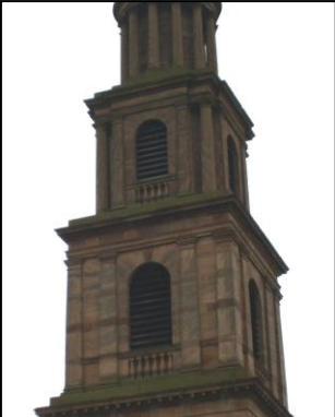
Antennas hidden behind GRP louvers made to match the exiting louvers exactly
