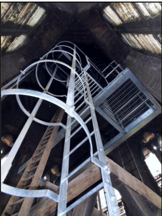
Typical view of a ladder installed to provide safe access through a church tower
