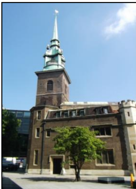
Antennas hidden behind GRP louvers made to match the exiting louvers exactly
