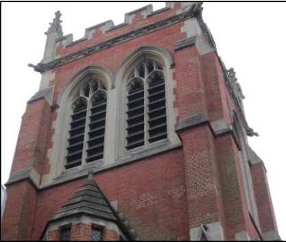
Antennas hidden behind GRP louvers made to match the exiting louvers exactly
