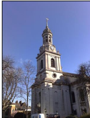
Antennas hidden behind GRP louvers made to match the exiting louvers exactly
