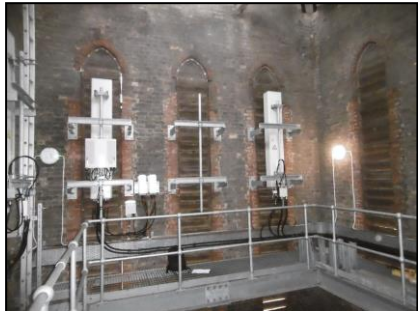
Antennas hidden behind GRP louvers made to match the exiting louvers exactly
