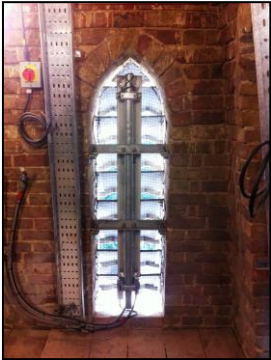
Antennas hidden behind GRP louvers made to match the exiting louvers exactly
