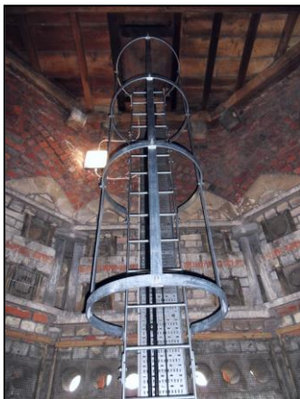
Typical view of a ladder installed to provide safe access through a church tower
